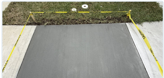
4 Finished sidewalk replacement with broom finish and safety controls.
