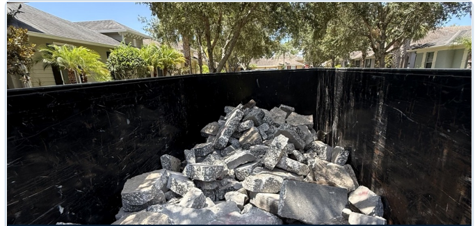
2 Concrete debris removed and hauled off site during demolition.
