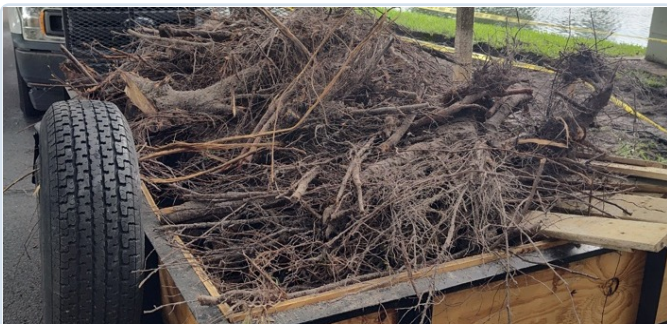
3 Removed roots and vegetation staged for proper disposal.
