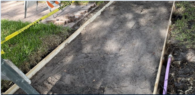
1 Prepared and formed replacement area prior to concrete placement.
